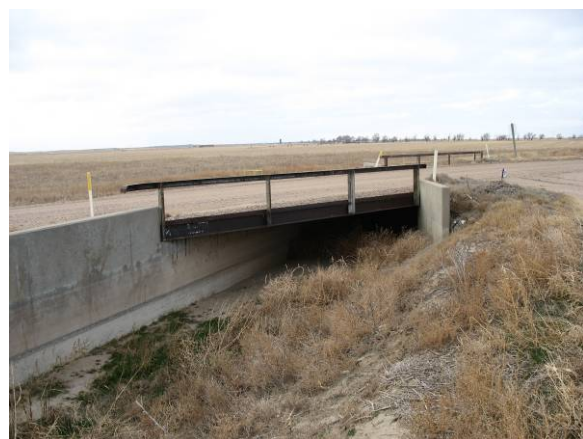
Figure 3.3 Typical County Road Bridge
