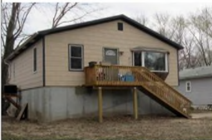
Construction on crawlspace
