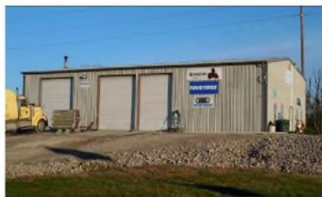
Elevation on compacted fill
