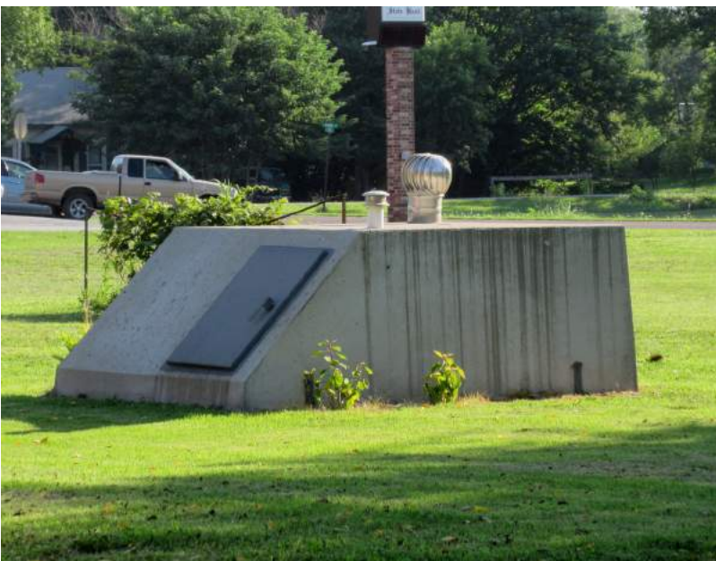
In-Ground Storm Shelter
