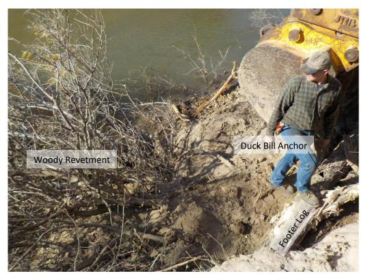
Figure 3. Woody Revetment Installation on the Lower Smoky Hill River, Kansas.
