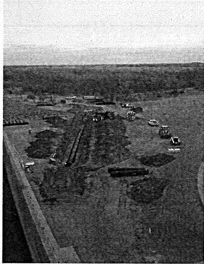
Winter 2016/2017 – 700 LF of Naponee Irrigation Conduit Was Replaced & New Lined Slots for Irrigation Stoplogs and Trash Racks Were Constructed
