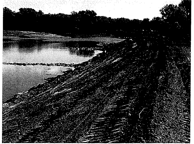
Completed stream restoration site
