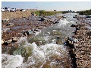
California's Budiselich Dam fishway
