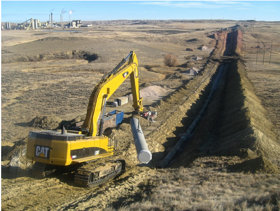
Photo 6 - Example of water transmission line construction and installation
