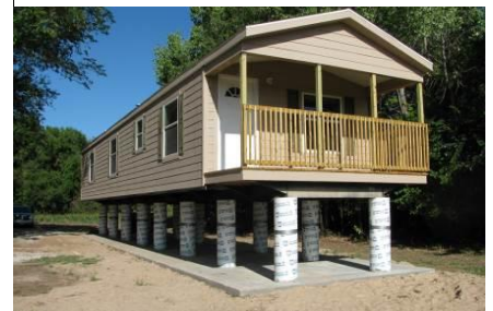
Elevation on post, piers, etc.
