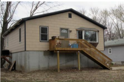
Construction on crawlspace
