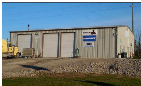
Elevation on compacted fill
