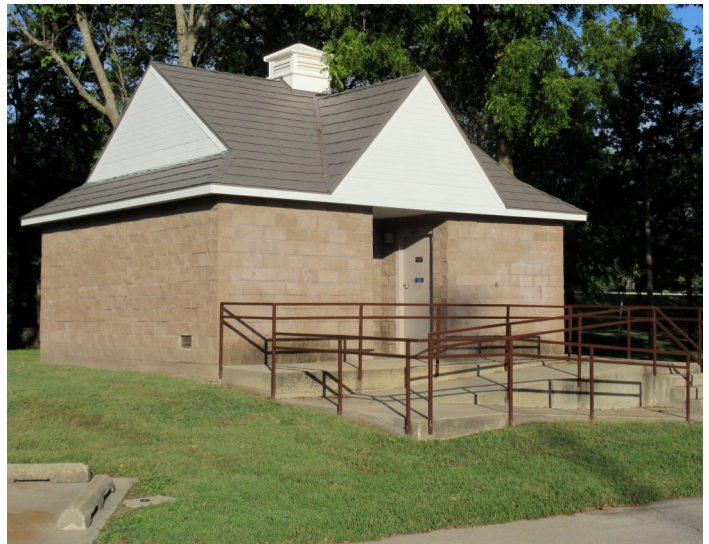
Above : This park restroom is properly elevated on fill and withstood a flood without damage.
