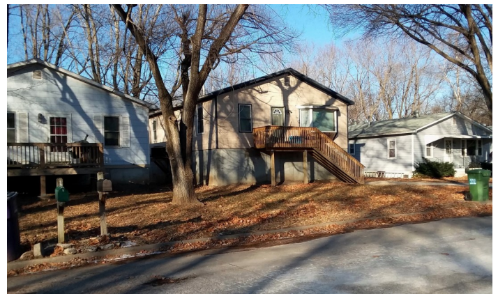
Above: Three homes that demonstrate the value of elevation with freeboard for insurance purposes and the value of mitigation as well.
