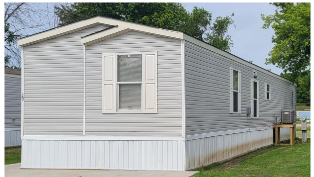
Manufactured home properly anchored and elevated utilities
