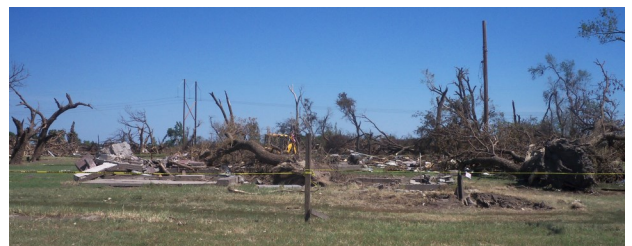
Substantially damaged structures
