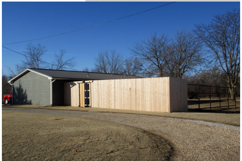
Above: This privacy fence in the Special Flood Hazard Area (SFHA) needs a local floodplain permit and potentially a state floodplain permit.
