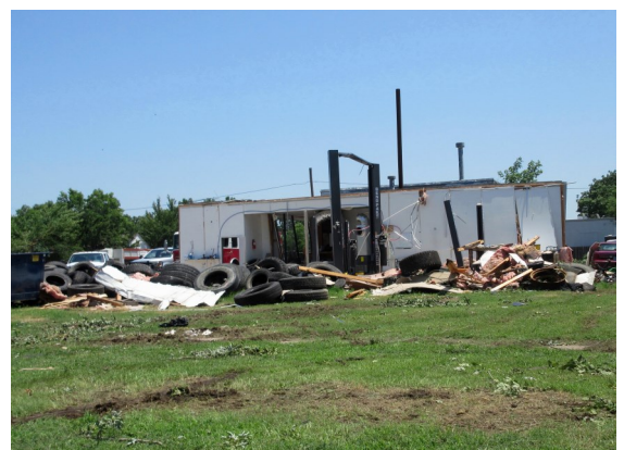
Above: This repair shop in Eureka suffered tornado damage in 2018.
