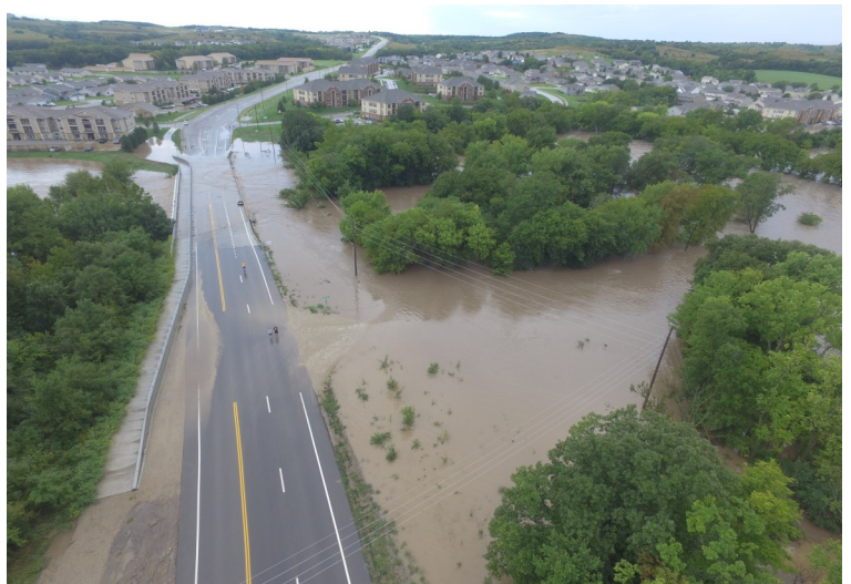
Above: Water approaches apartment homes in Manhattan during the Labor Day 2018 flood event.
