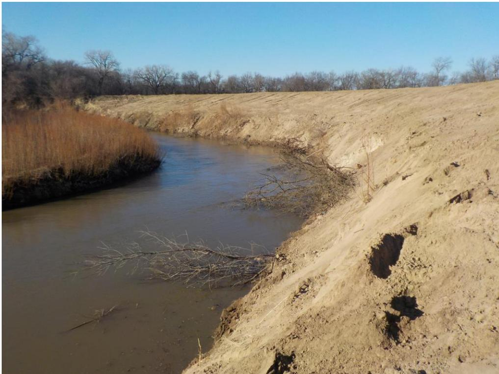
*Figure 1. Example of Woody Revetments and Bank Shaping following construction on the Smoky Hill River, Kansas (Site 27, January 2017).*
