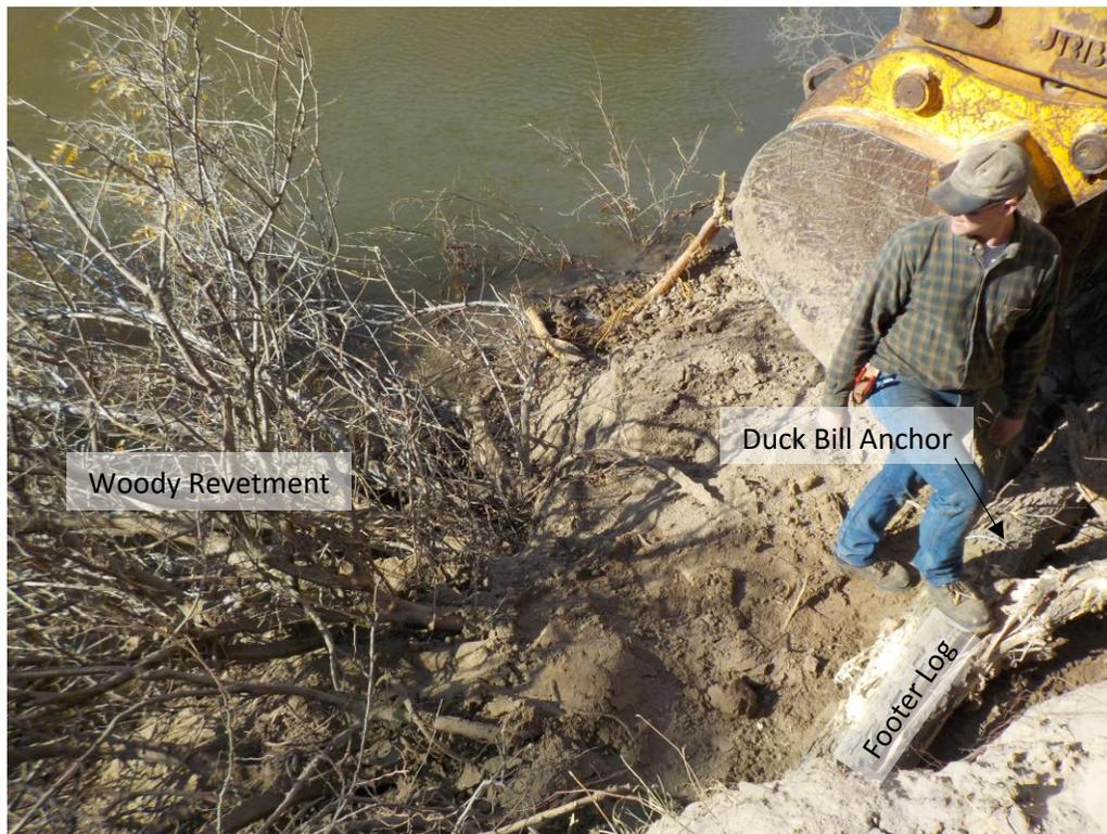
Figure 3. Woody Revetment Installation on the Lower Smoky Hill River, Kansas.
