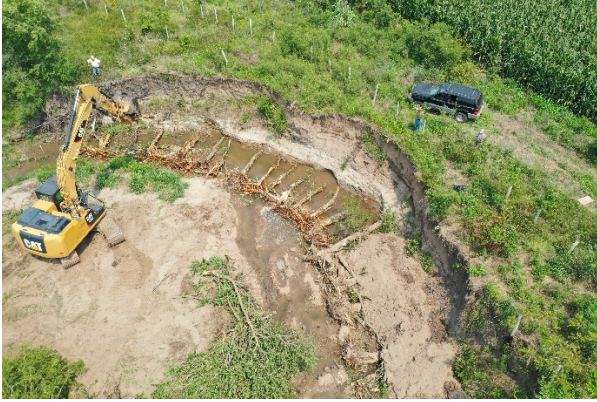
Bank stabilization using rootwads.
