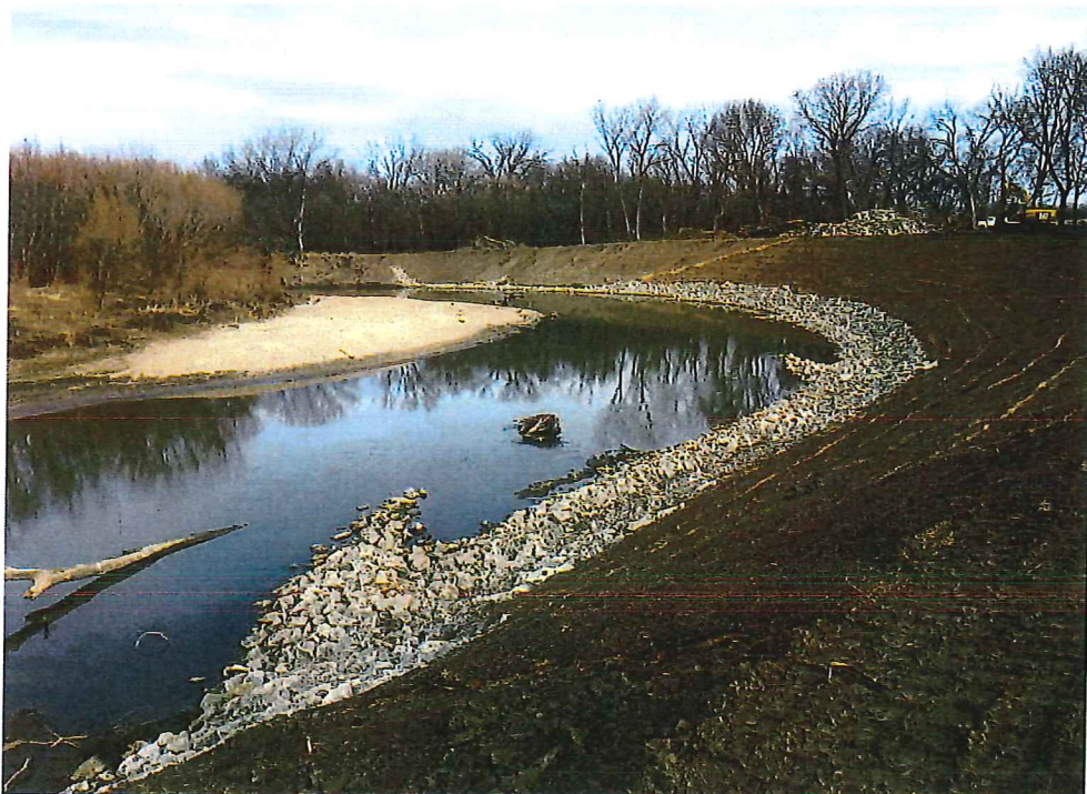
Cottonwood Site 15 project - construction completed in January.
