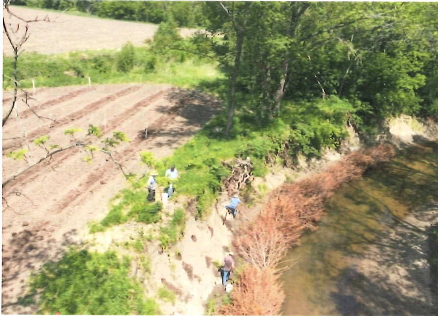
Photo: The simplest kind of project our Forestry RCPP may support. Immediate bank stability is achieved by anchoring large dead trees and live willow cuttings along the toe of the bank, while long-term bank stability will be ensured by the hardwood trees planted along the edge of the field.
