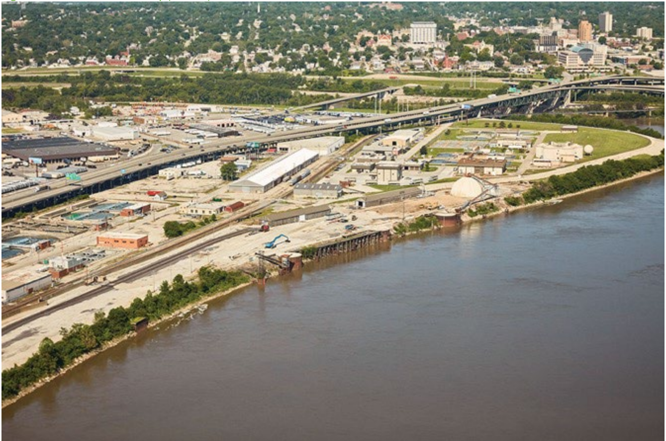
Figure 168. Port of Kansas City (PortKC)
