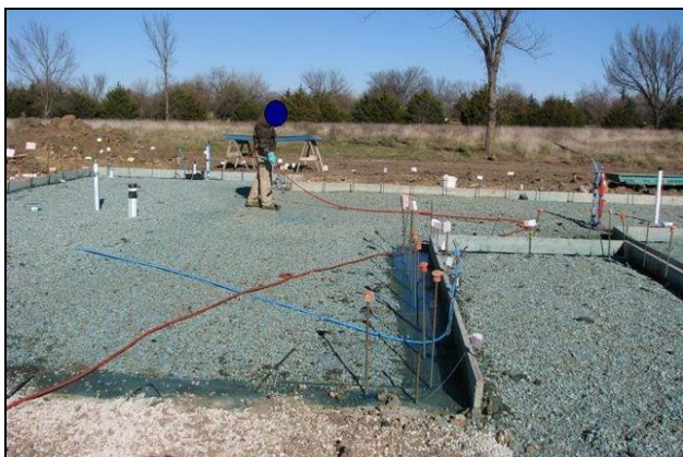
Above: After the interior final grade is established, the applicator applies termiticide to the flat surface over which cement will be poured.
