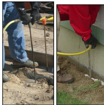
Far left: The applicator completes the interior vertical application before the flat concrete surface is poured.
